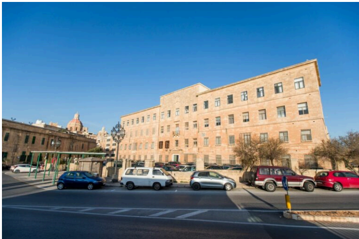
The Evans Building site. Photo: Malta Strategic Partnership Project via Facebook
